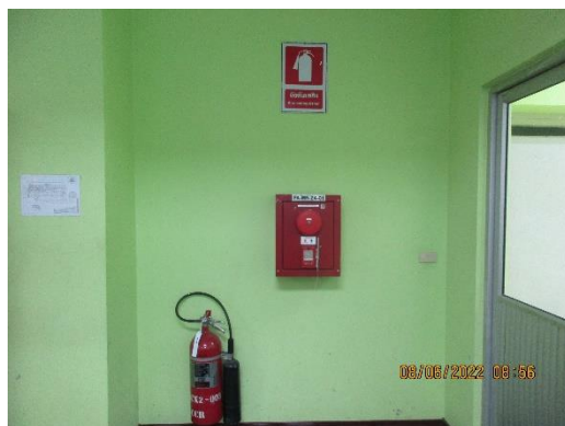
Manual Fire Alarm & Fire Extinguisher
